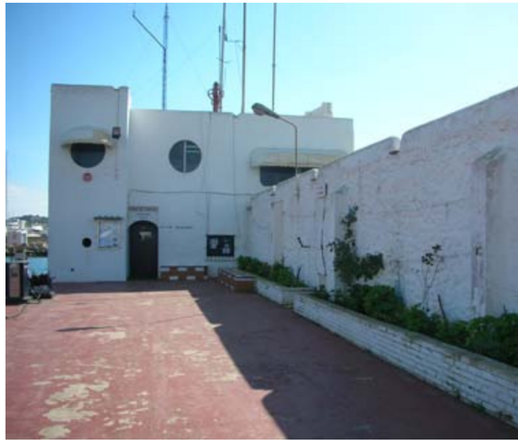
RECEPCIÓN ANTES / RECEPTION BEFORE
