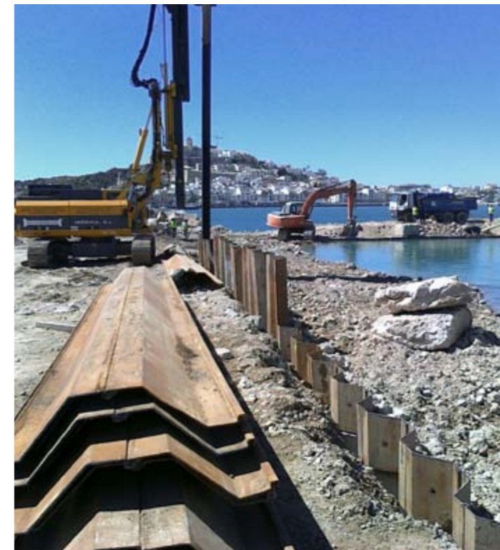
DIQUE EXTERIOR ANTES / OUTER DOCK BEFORE
